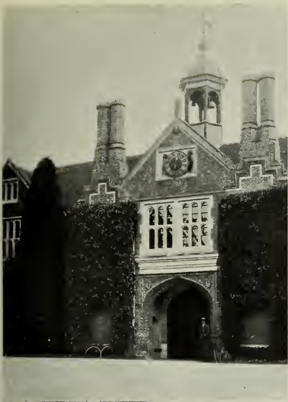
Entrance in West Front.
